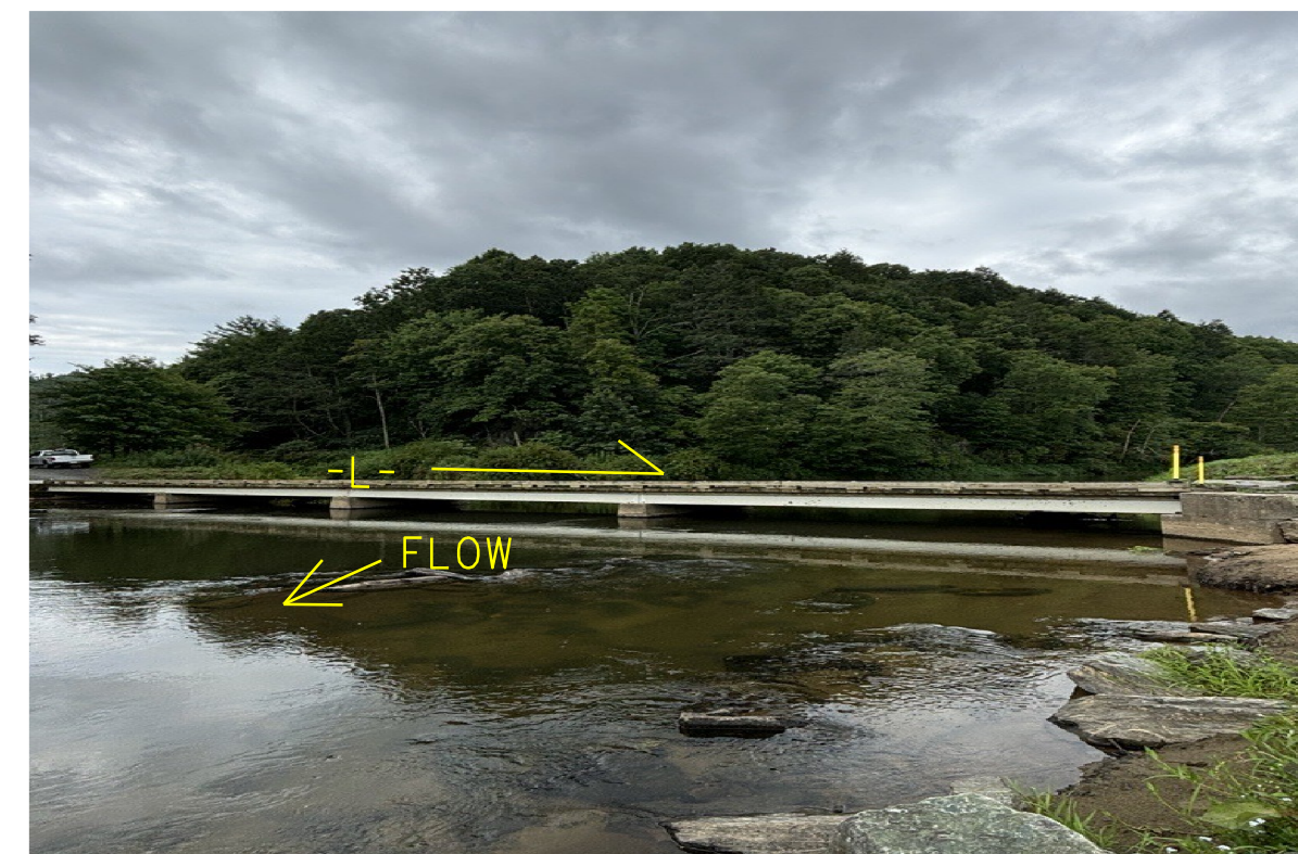
PHOTO #4: DOWNSTREAM OF EXISTING BRIDGE.
