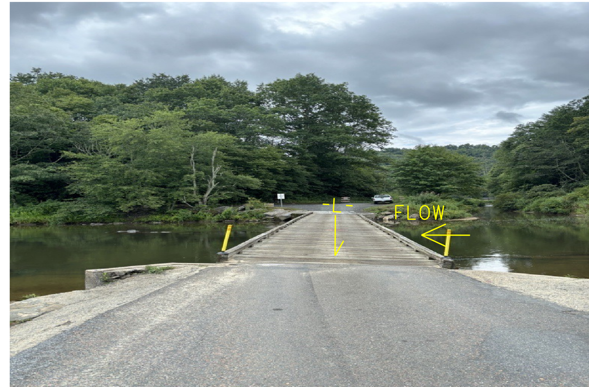
PHOTO #2: END BENT NO. 2 OF EXISTING BRIDGE LOOKING SOUTH EAST (DOWNSTATION).
