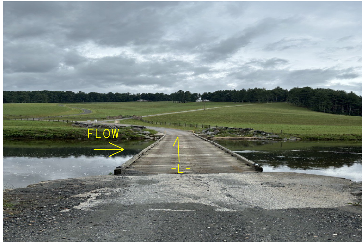
PHOTO #1: END BENT NO. 1 OF EXISTING BRIDGE LOOKING NORTH WEST (UPSTATION).
